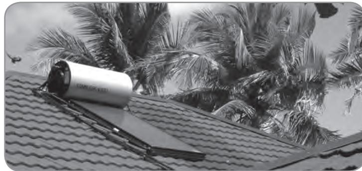
Active solar systems use special solar collectors that look like boxes covered with glass. Dark-colored metal plates inside the boxes absorb the sunlight and change it into heat. (Black absorbs more sunlight than any other color.) Air or a liquid flows through the collectors and is warmed by this heat. The warmed air or liquid is then distributed to the rest of the house just as it would be with an ordinary furnace system.
