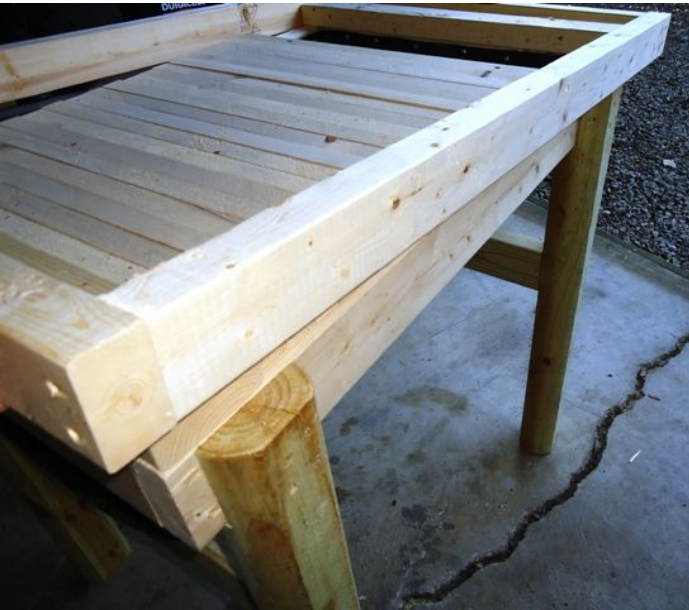
Step 43: Good view of the roof frame at rest on the legs.
