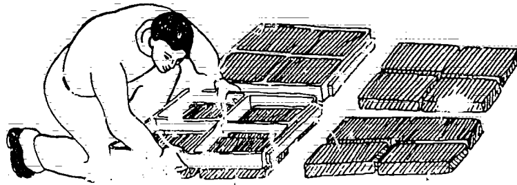
Figure 41. Lifting the forms from freshly made blocks.
