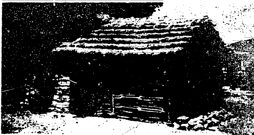
Figure 4. The right half of this residence in Greece shows the wattle in place. Daub will follow.
