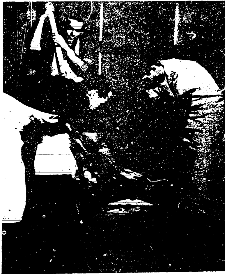
Figure 54. Charging mold box with soil mix.
