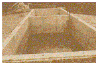
Figure 8. Structure for soaking logs.
